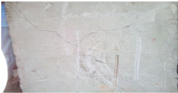
cracks on conventional slab
